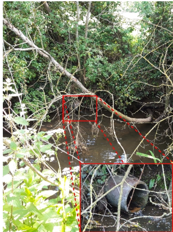
Photograph 10 – Highway drain outfall into Poulton Brook
