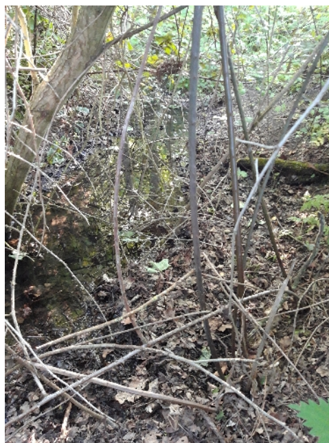
Photograph 4 – Drain C at the right angle bend
