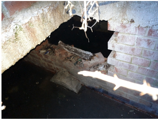
Photograph 5a - Inside the manhole
