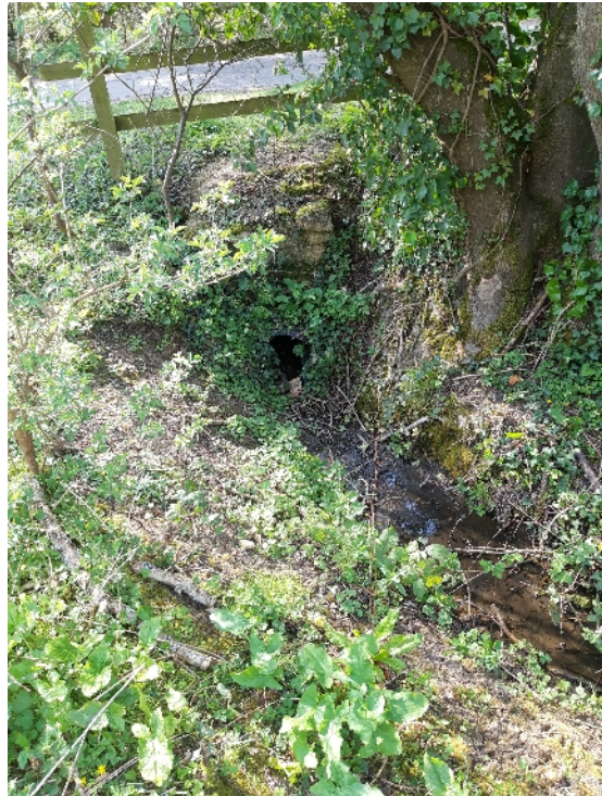
Photograph 7 - Drain E Looking back to Oak Road
