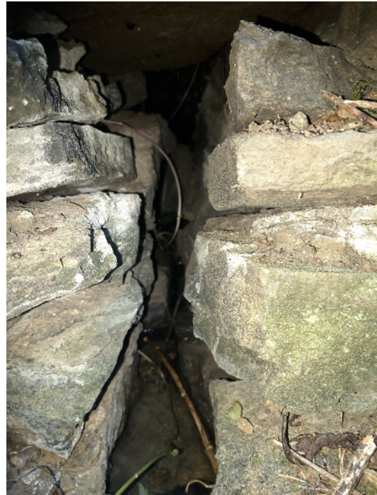
Photograph 12 – Inside the dry-stone outfall
